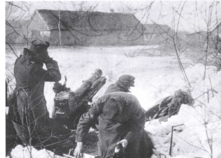
Gebirgsjager troops fire a 7.5cm Geb36 gun. Firing an artillery piece in the snow could be frequently problematic for the gun crew. The recoil would regularly drive the weapon deep into the snow and would often cause inaccurate firing. For this reason this 7.5cm Geb36 gun has been modified – its wheels have been removed and replaced with sturdy gun trails.
