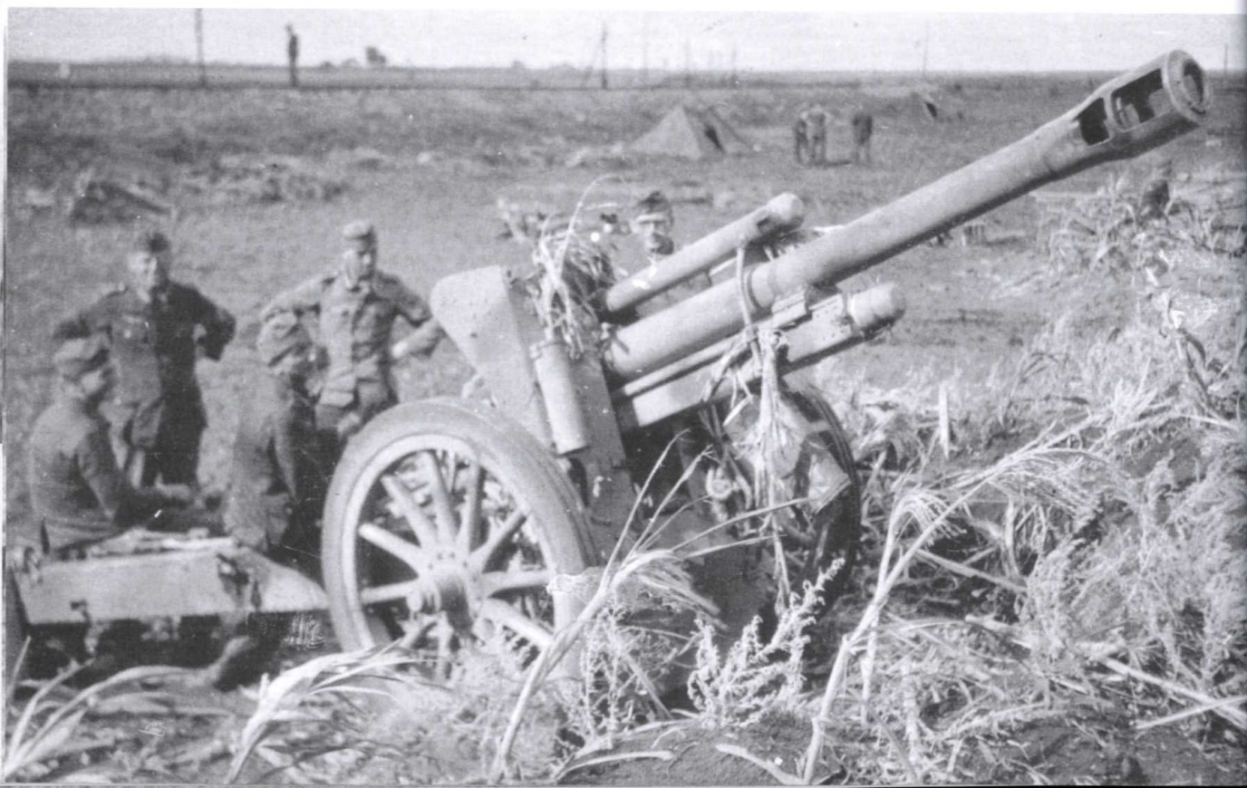
Two photographs showing the gun crew of a modified 10.5cm le FH 18/42, preparing to fire the gun in anger. The 10.5cm was the standard light artillery piece deployed in the artillery divisions on the Eastern Front. However, in order to give the gun better punch on the battlefield the weapon was modified in 1942. The barrel was lengthened, a cage muzzlebrake was fitted, and the carriage was a lightened version of the le FH 18 design.
